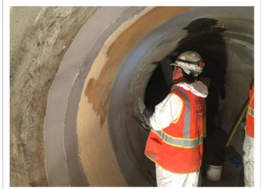
Interior Joint Grouting
