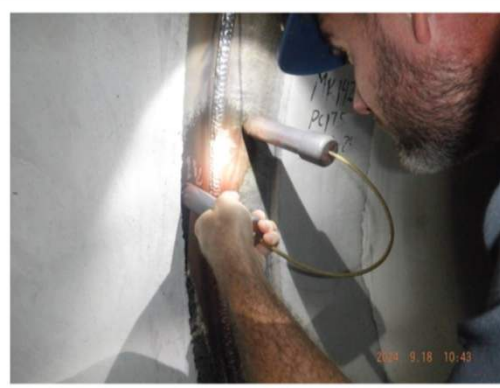
Weld Magnetic Particle Testing
