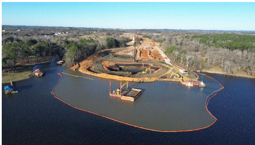
Aerial view of Lake Palestine Pump Station and dredge activities, April 2024
