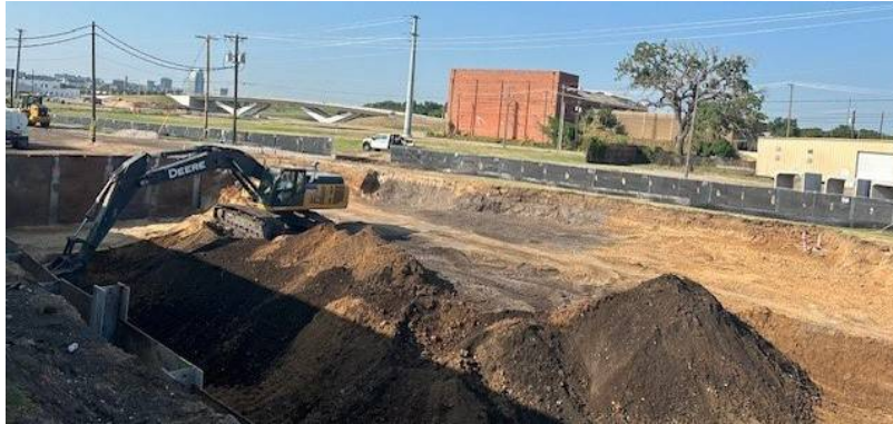
The District's operations yard environmental cleanup
