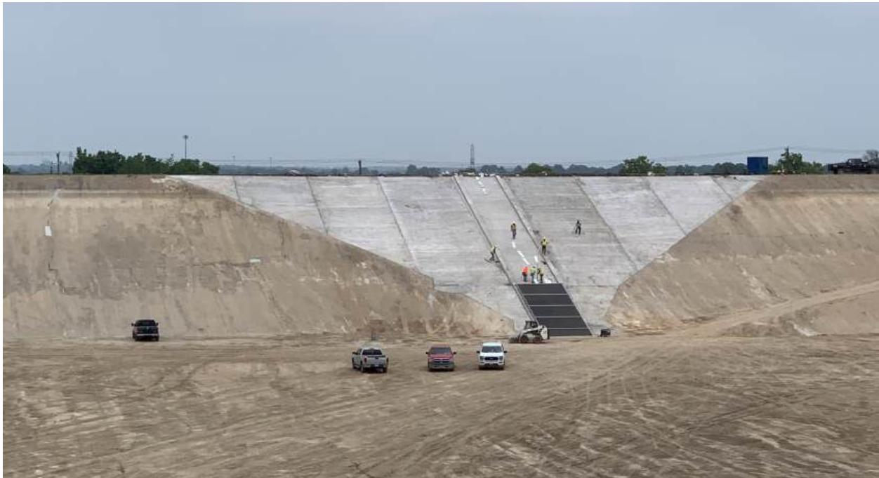
Kennedale Balancing Reservoir (Phase 3) - Construction of Cell 2 Outlet, March 2024
