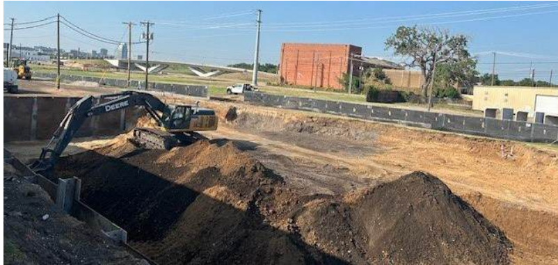
The District's operations yard environmental cleanup
