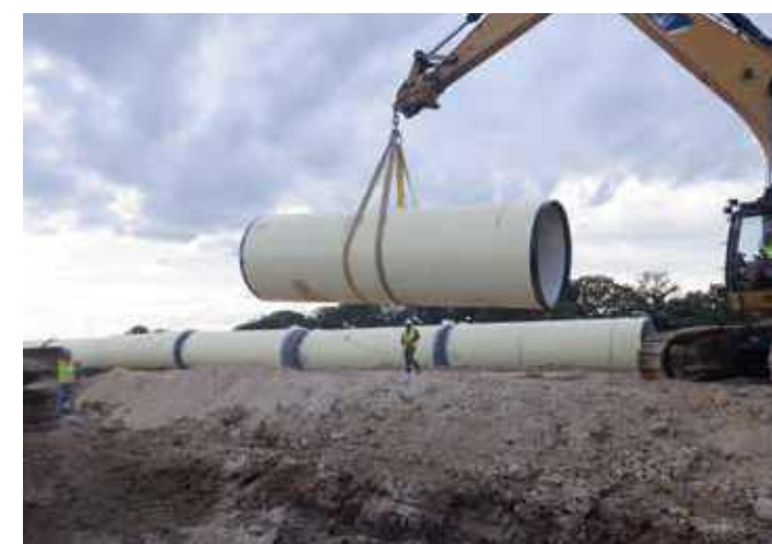
PL19TUN Preparing to install open-cut pipe joint
