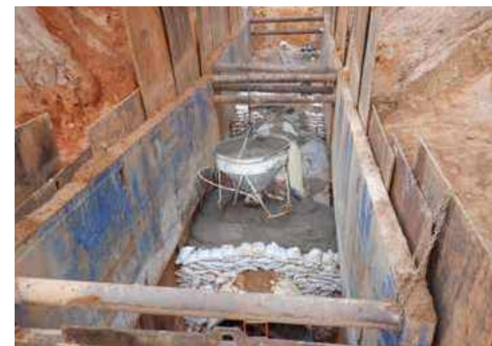
PL19TX Placing flowable fill encasement near FM315
