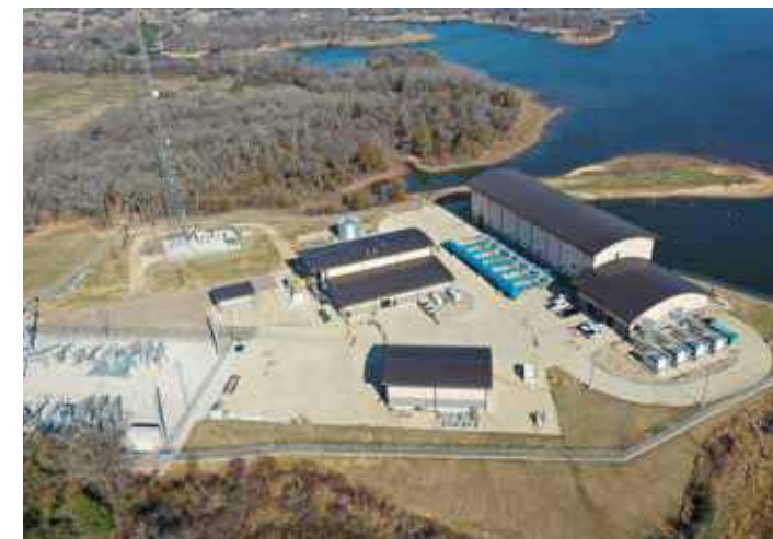
JCC1 Aerial photo of completed facility structures
