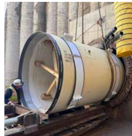
PL19TUN Royal Blvd Tunnel Pipe Installation
