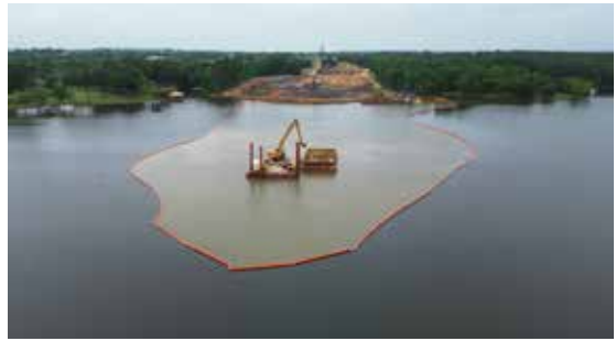
LP1IN Dredging Activities in the Intake Channel
