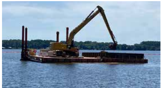
LP1IN Dredging Sediment from Intake Channel
