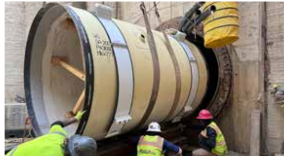
PL19TUN Royal Blvd Carrier Pipe Installation
