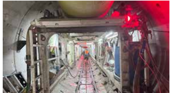
PL19TUN Back of TBM at Hollywood Lake Tunnel
