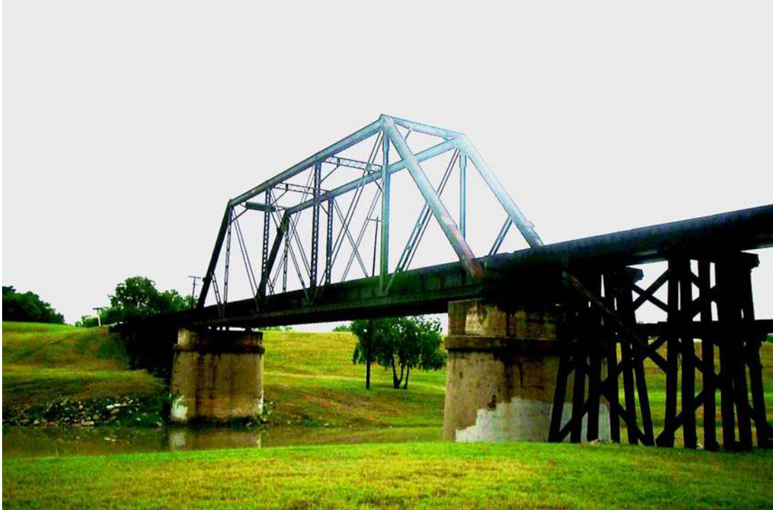
Figure 108. St. Louis, San Francisco and Texas Railway Bridge (Property Number 102).
