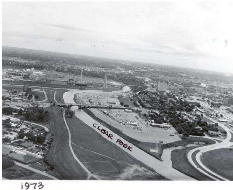
Figure 63. Original Clear Fork course, now serving as city drainage (photo courtesy of USACE, Fort Worth District).
