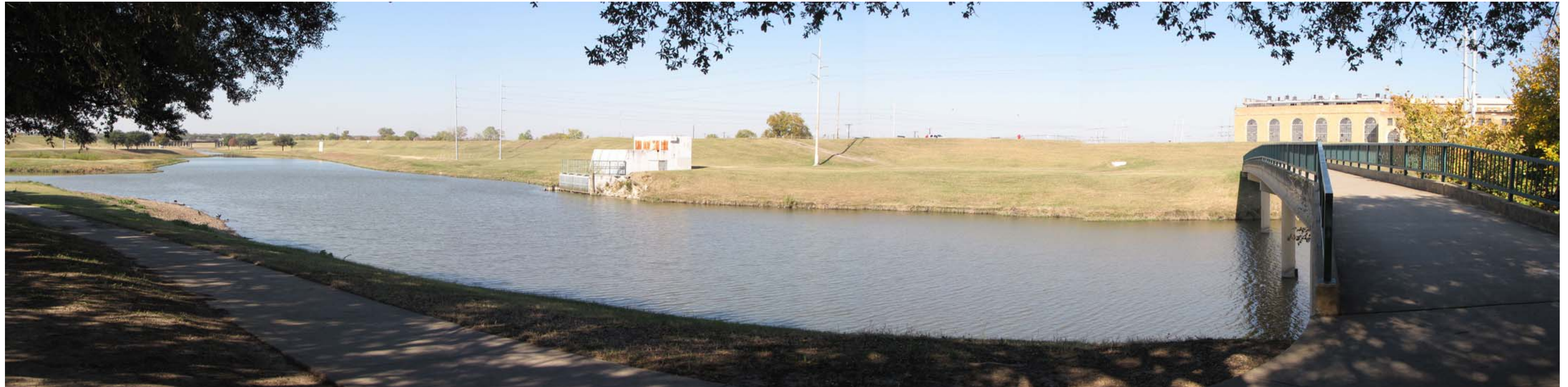
Figure 33. View looking north to the Fort Worth Power and Light intake station (Property Number 1-C) (photograph by Joseph S. Murphey).
