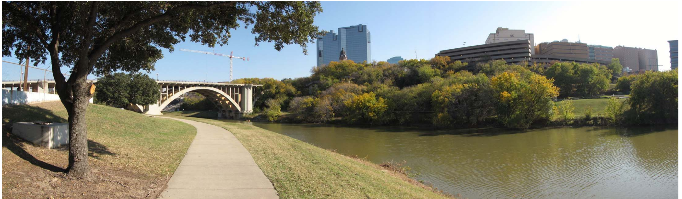
Figure 73. View looking east toward Paddock Viaduct (Property Number 103) (photograph by Joseph S. Murphey).
