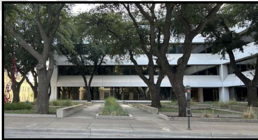
Figure 6 – USHealth Group Administration Building representative of the Late Modern Style (alternative style design) (Built c. 1975)
