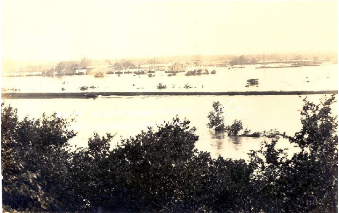
Figure 50. Looking toward North Main Street from Samuels Avenue during 1922 flood (photo courtesy of USACE, Fort Worth District).
