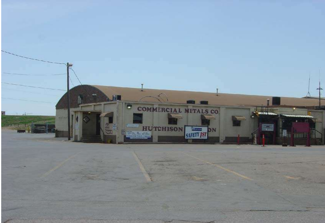
Figure116. Hutchinson Pipe & Waste Material Company, 601 North Throckmorton (Property Number 13).
