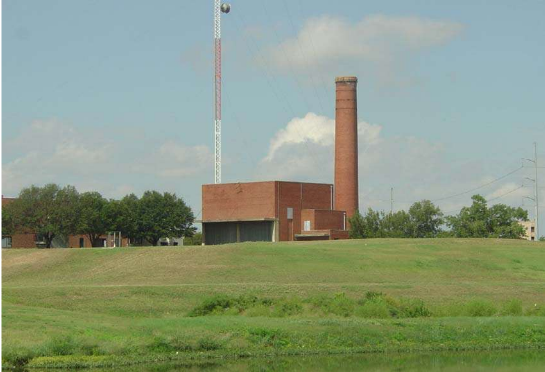
Figure 127. Former city of Fort Worth incinerator, 900 Woodward (Property Number 96-A).
