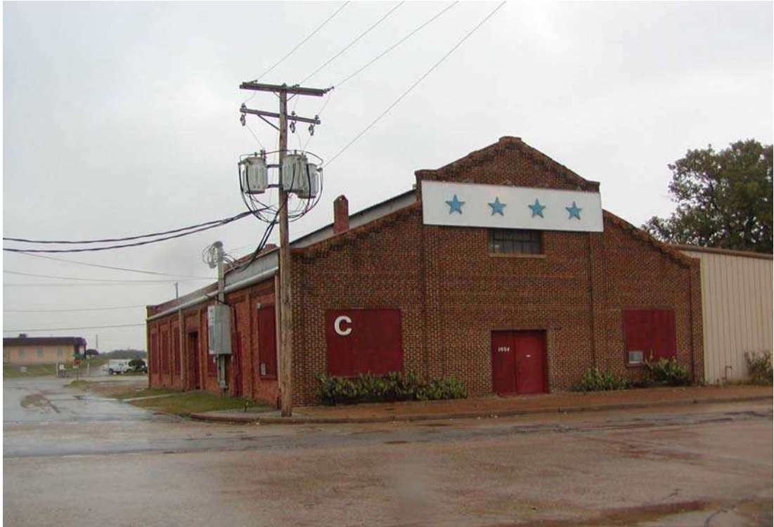
Figure 96. 1024 North Commerce Street (Property Number 64).
