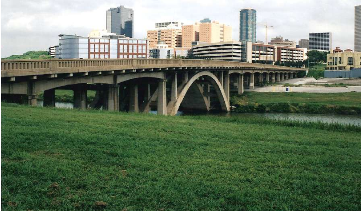
Figure 107. Henderson Street Bridge (Property Number 101).
