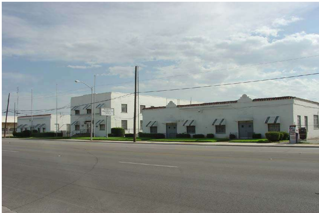
Figure 38. Panther Oil and Grease Manufacturing Company buildings at 832, 840, 842 North Main Street (now Texas Refinery Corporation) (Property Number 50 A-C).
