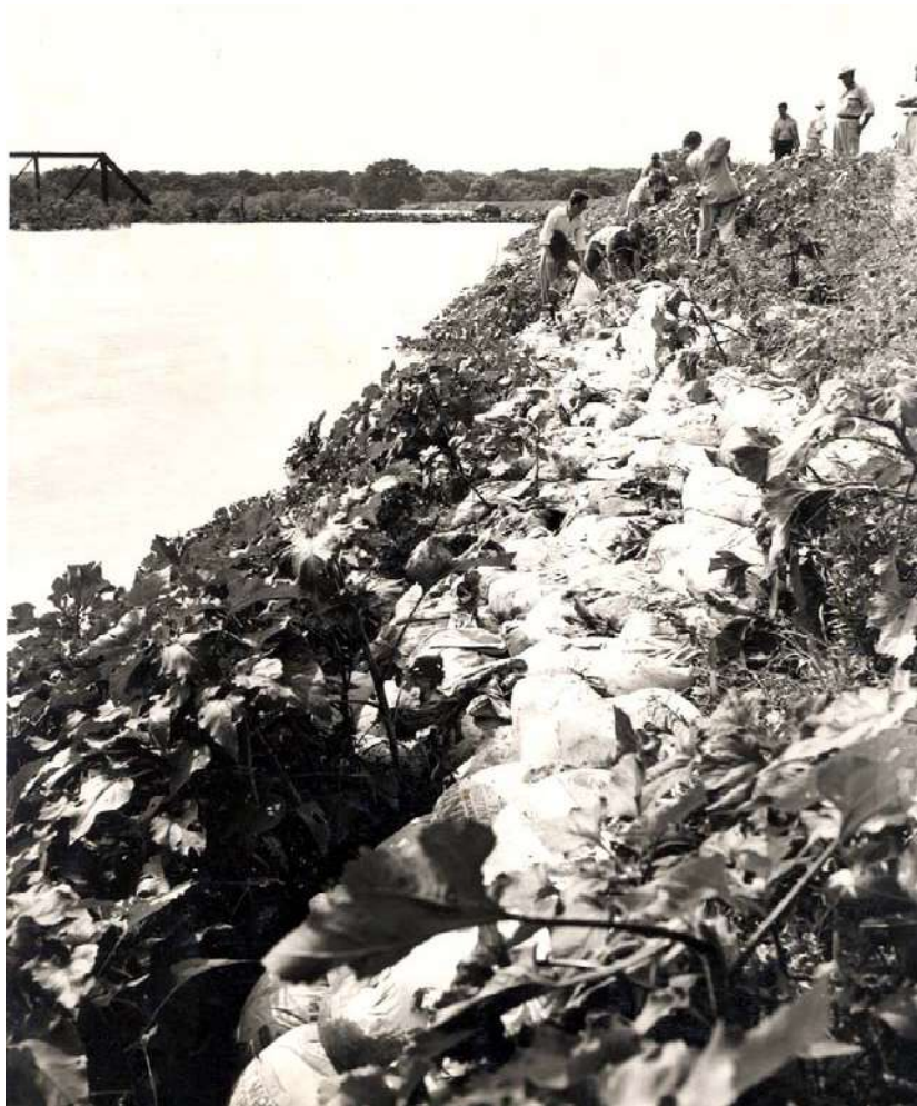
Figure 58. Sandbagging at North Main Levee on east side of West Fork, May 1949, looking northwest (photo courtesy of USACE, Fort Worth District).
