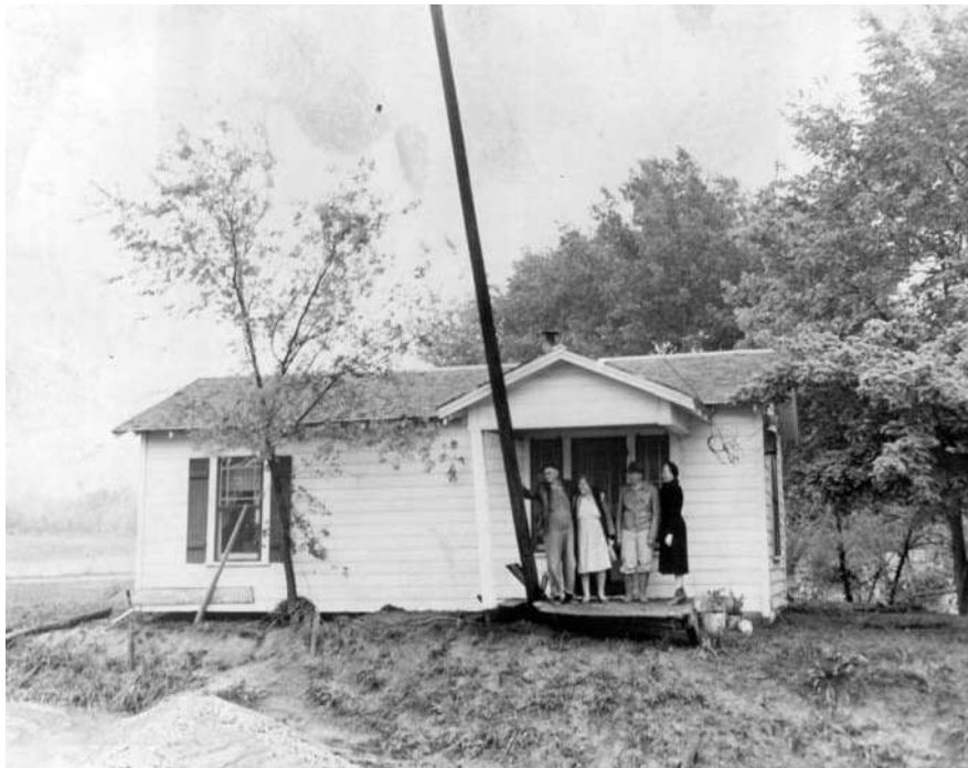
Figure 23. Photograph from 1942 flood. Caption reads, "House in North Fort Worth completely washed away from foundations by Trinity flood" (photo courtesy of USACE, Fort Worth District).
