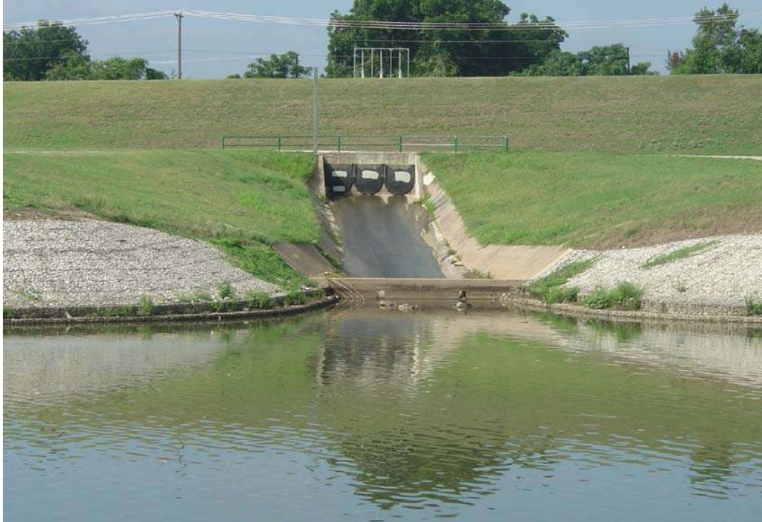
Figure 66. Sluice at the TRWD Dam.
