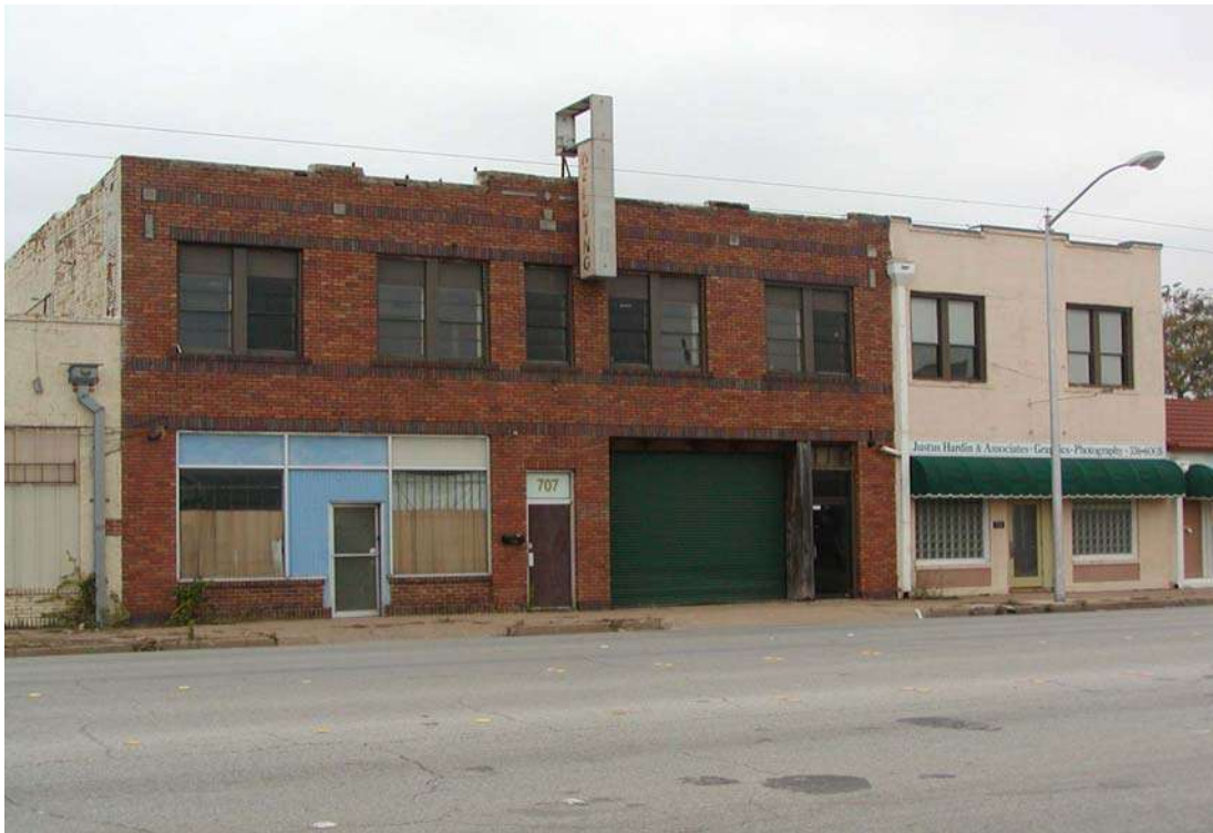
Figure 93. 709 North Main Street (Property Number 25).
