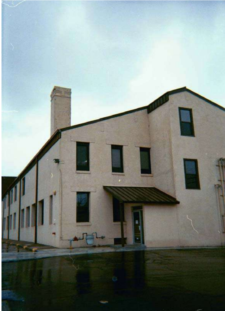
Figure 39. Former Magnolia Oil facility at 528 North Main Street (Property Number 11).
