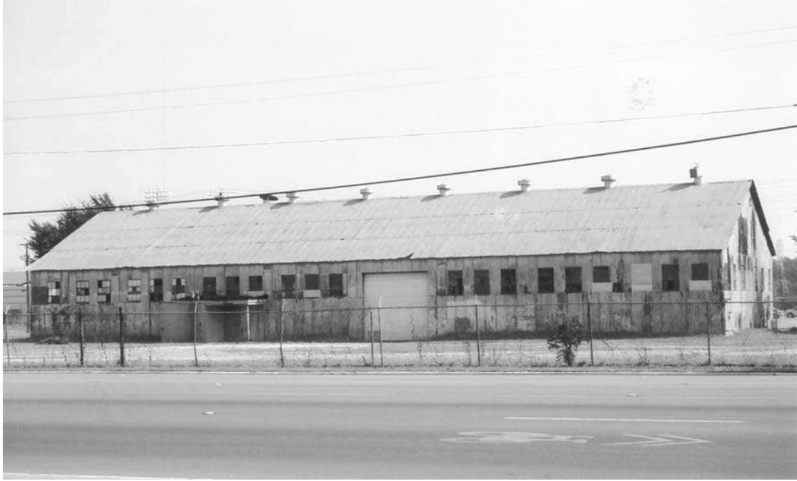
Figure 95. 625 North Commerce Street (Property Number 15).
