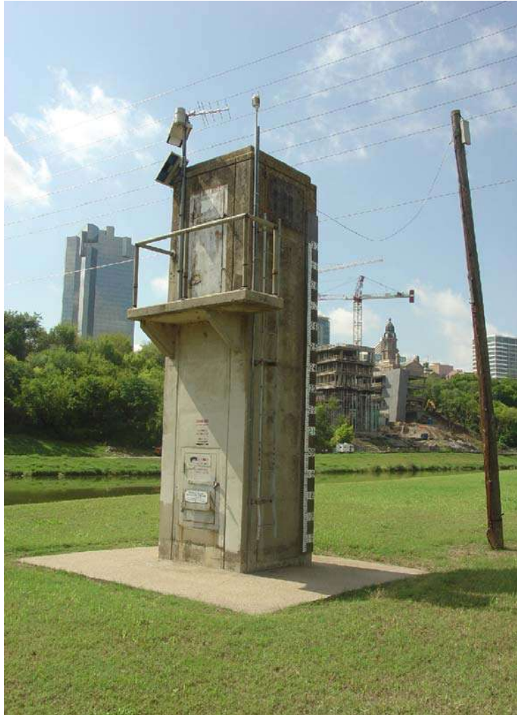
Figure 69. U.S. Geological Survey gauging station at Nutt Dam.
