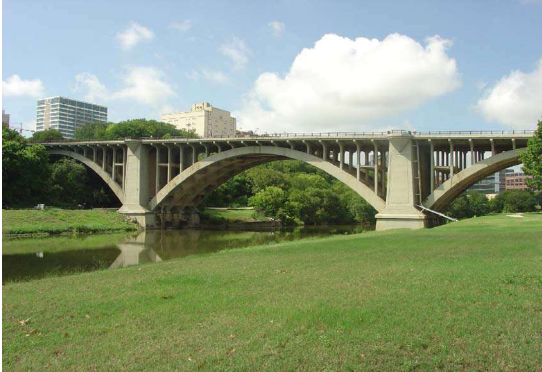
Figure 88. Paddock Viaduct (Property Number 103).
