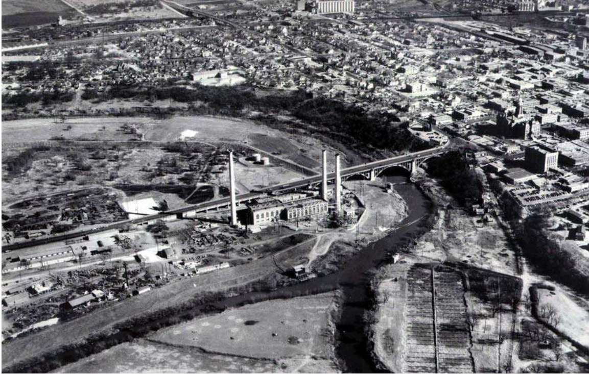
Figure 31. 1950 aerial view with TXU power plant in foreground (photo courtesy of USACE, Fort Worth District).
