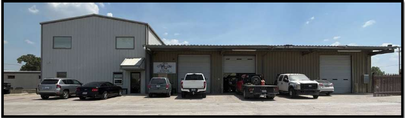
Figure 7 – Texas Towing Warehouse on South Commercial Street representative of the Modern Industrial Style (built c. 1972)
