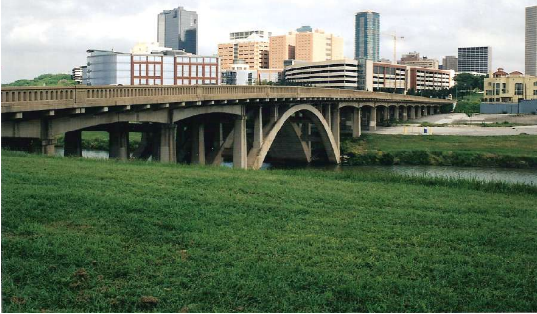
Figure 89. Henderson Street Bridge (Property Number 101).
