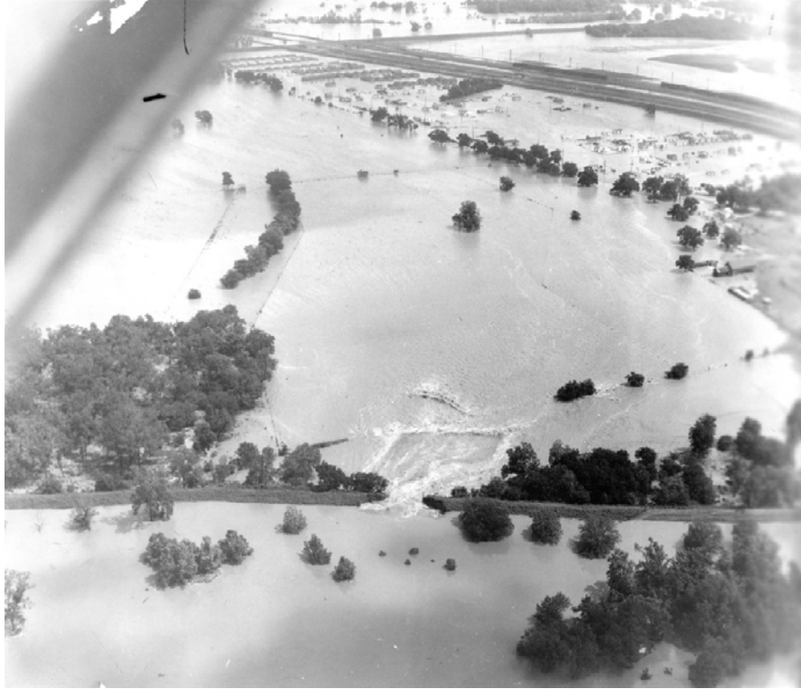
Figure 57. Levee break in Lower West Fork Levee, May 1949, looking northeast (photo courtesy of USACE, Fort Worth District).
