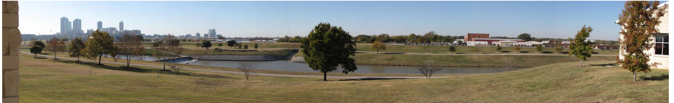
Figure 72. View looking southwest toward the TRWD Dam and the levee system (Property Number 104) with former Pier 1 building to left in background (photograph by Joseph S. Murphey).
