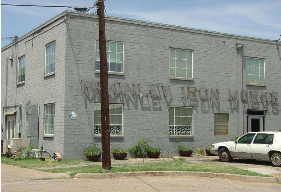
Figure 40. McKinley Iron Works at 901 North Throckmorton Street (Property Number 47).
